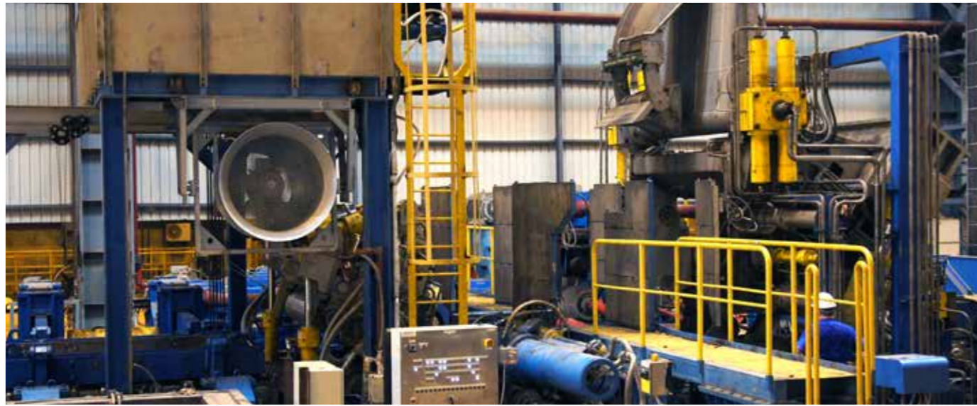
Coil box in open position
